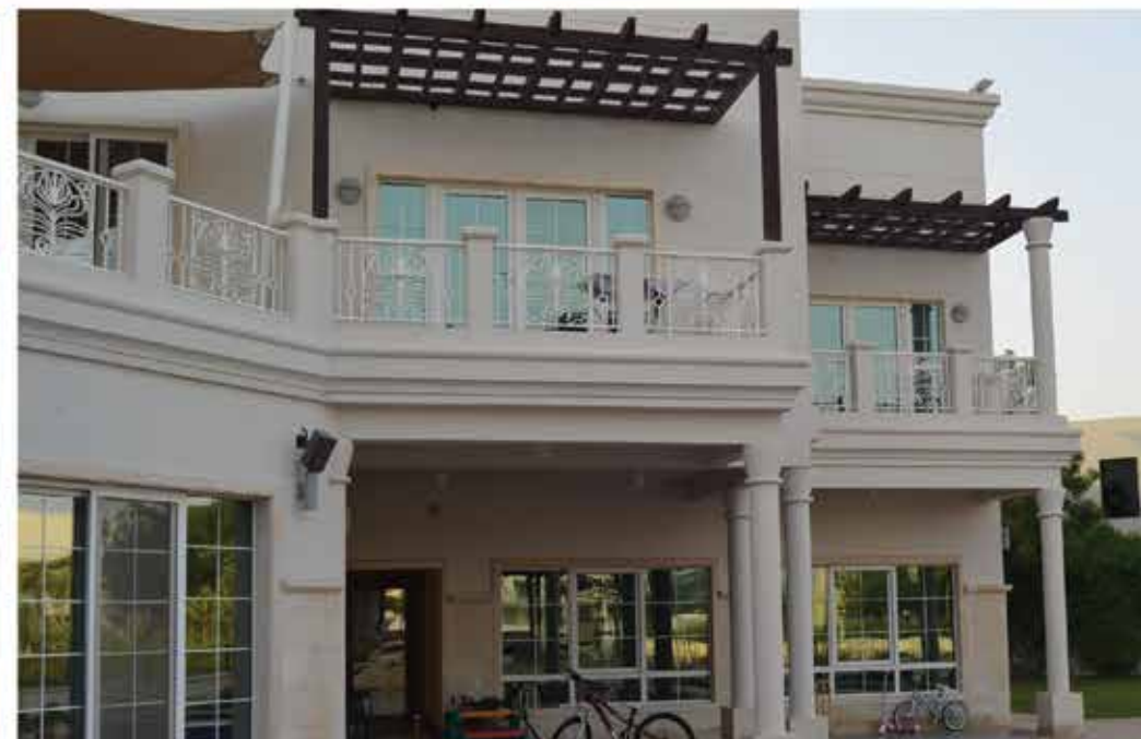
VILLA INTERIORS, EMIRATES HILLS, DUBAI
